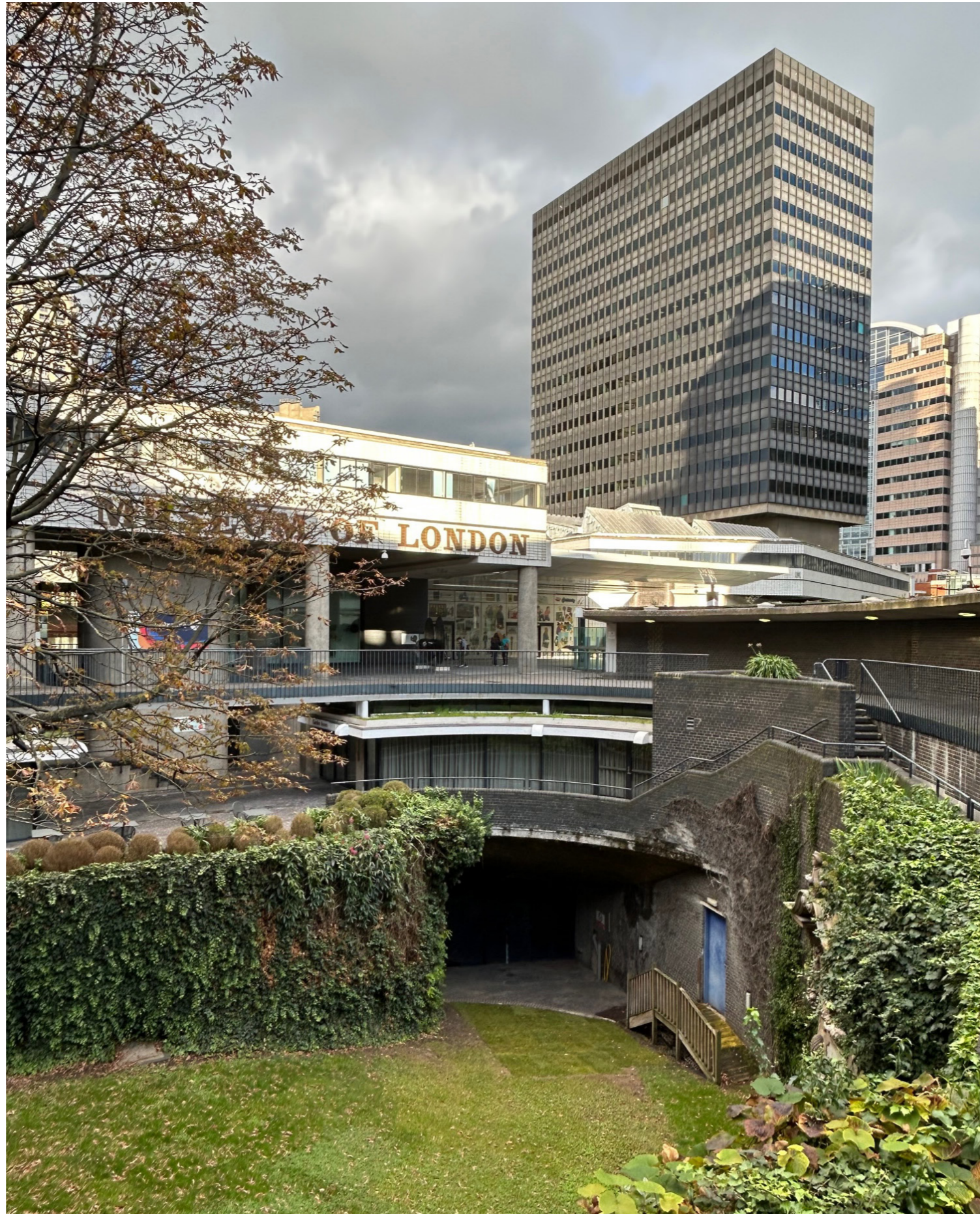
Photo: Existing highwalk level view looking over the Rotunda garden onto the Museum of London with Bastion House to the right of the image
