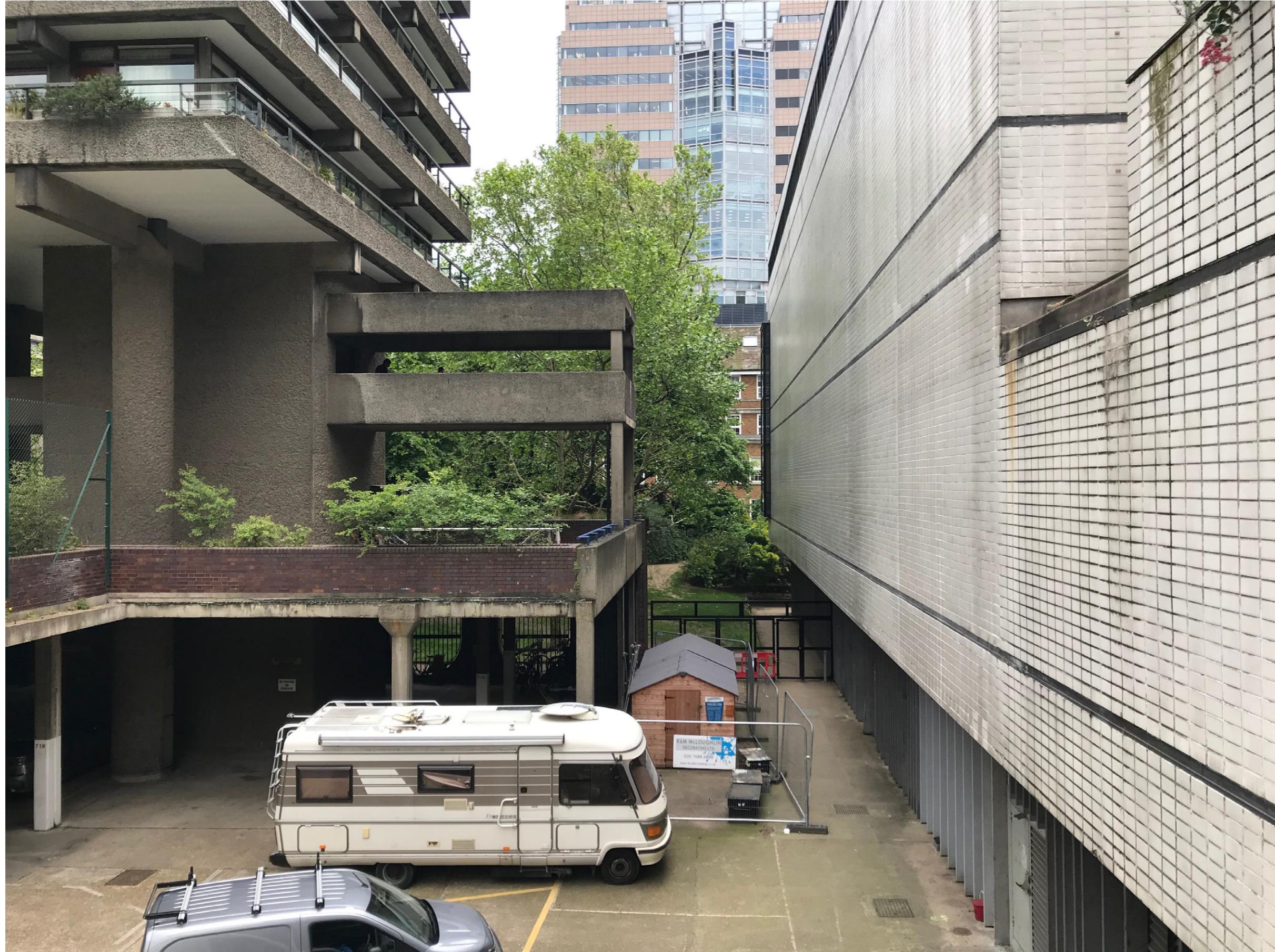
Photo: Existing view of Service Yard and Mountjoy House Highwalk dead-end
