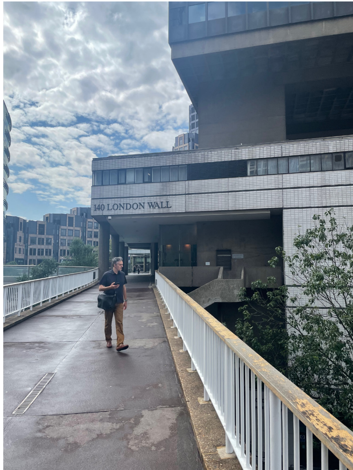
Highwalk route from the east
