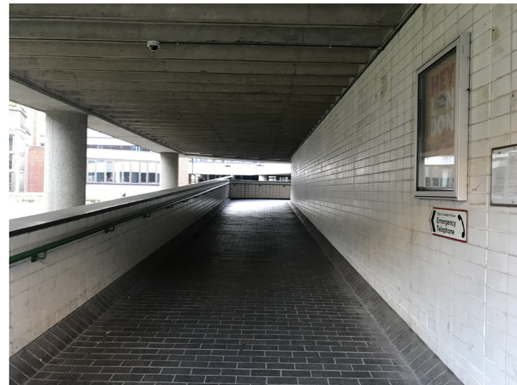
Highwalk route from the north
